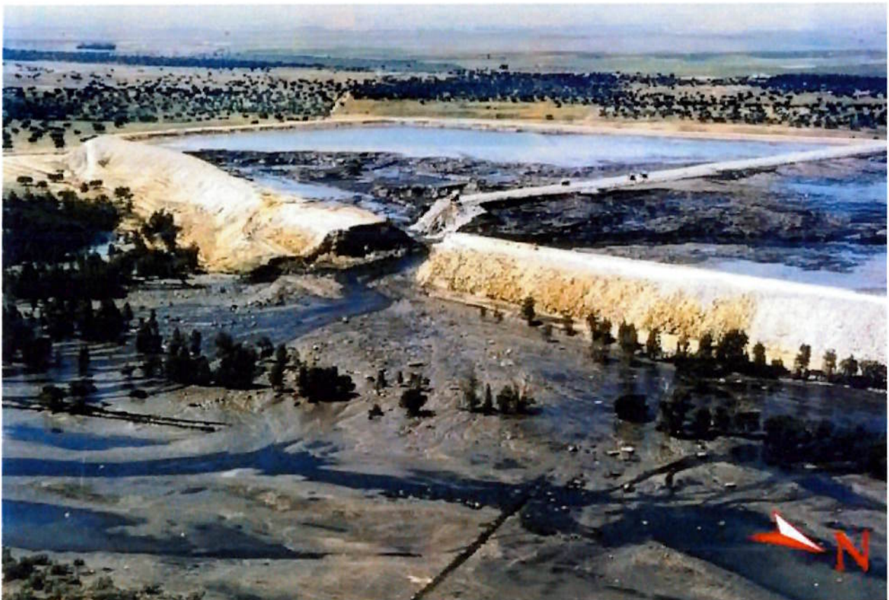
Figure 4 Los Frailes Tailings Dam Burst
