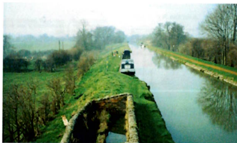
Figure 1 3 Canal embankment. Typically, water is retained by a lining. Although traditionally puddle clay was used for this purpose, replacement often utilises modern materials (courtesy British Waterways Technical Services)
